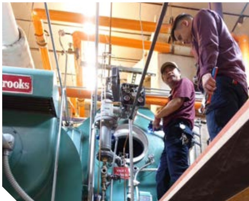
Local 302 Operating Engineers
