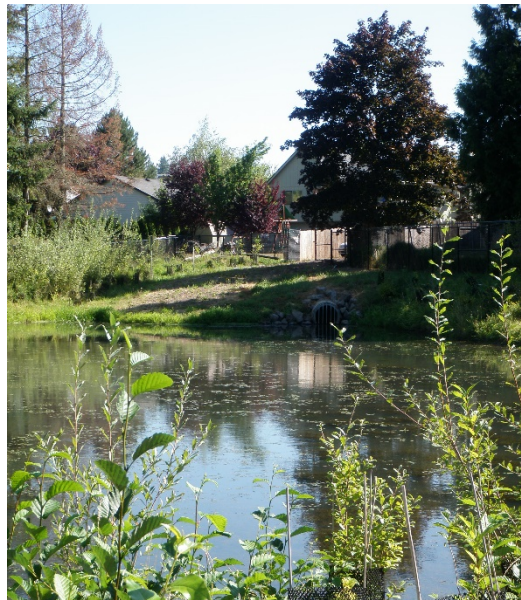
Figure 1. Encore Stormwater Facility
